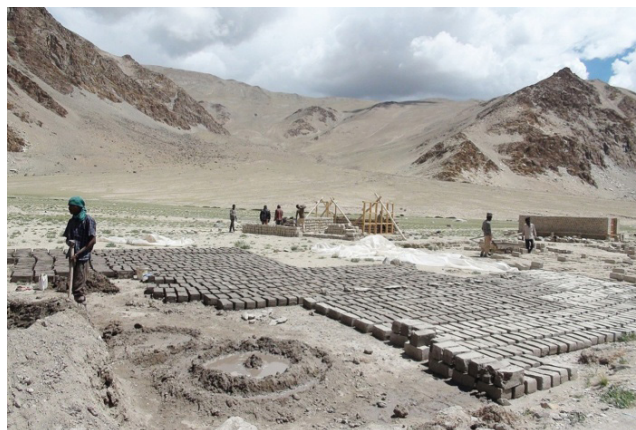
Figure 11. Construction work at near Puga wetlands.
